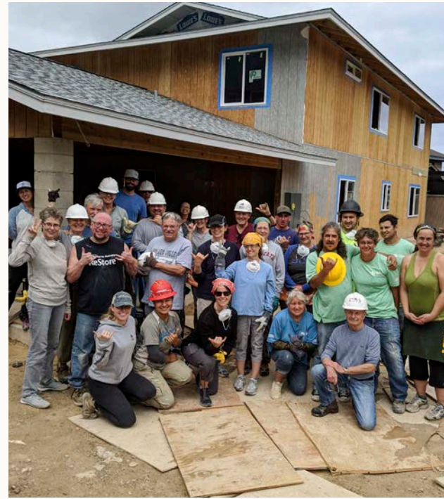
Above: Volunteers builders make a lasting impact by helping local families achieve their dream of safe, affordable housing. Photo credit: Hawai'i Habitat for Humanity
